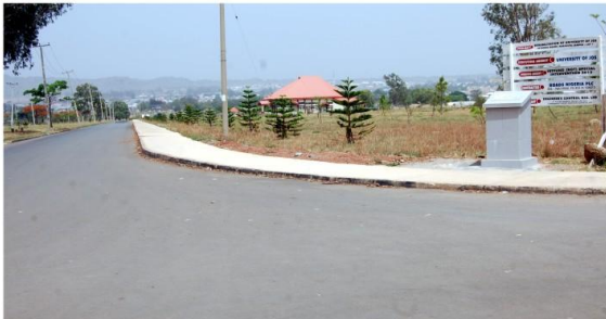
Newly completed Naraguta Campus Road network (1)
