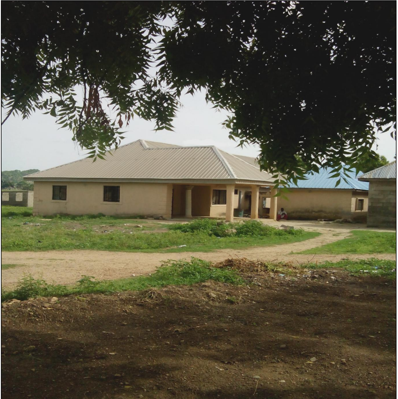
Plate 7: An Apartment being altered from the original plan at Shendam Low-Cost Housing Source: Field Survey (2014)
