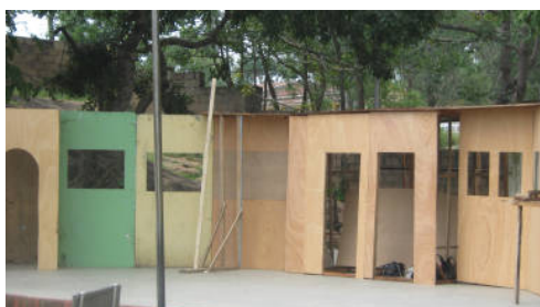
Plate vi: The stage after two days of work.
