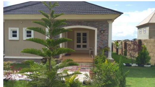
Figure 4: Porch on the south-east façade
