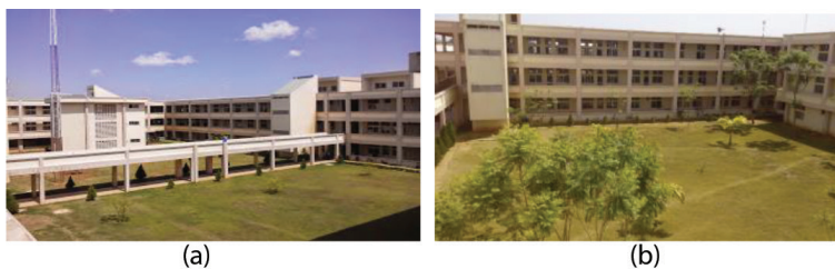
Figure 8. (a and b) Exterior views of Teaching Hospital complex.
