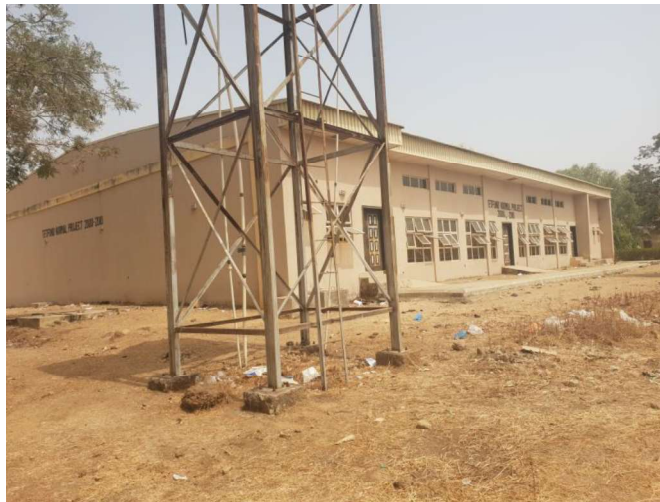
Figure 1: 500 Capacity Lecture Hall, Federal Polytechnic Bauchi Source: Authors 2021
