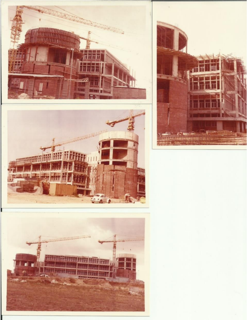
Figure 4: Progress of work on new library 1984
