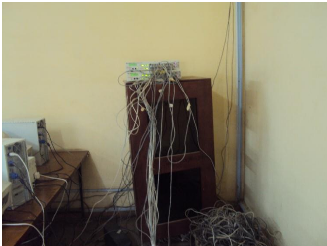
Figure 31: A criss- crossed network cable before the study. Courtesy ICT Directorate
